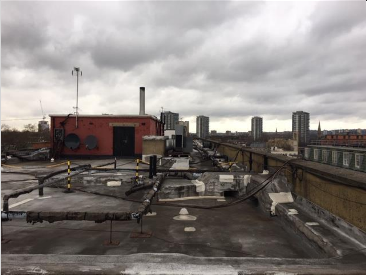
Roof level and existing plant
